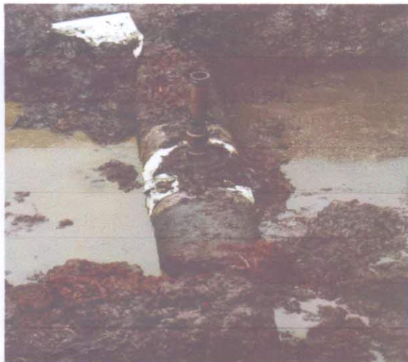
SPILL POINT AFTER EXCAVATION SHOWN: fig2
