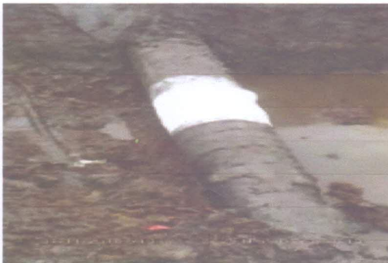
SPILL POINT AFTER REPAIRS: fig3
